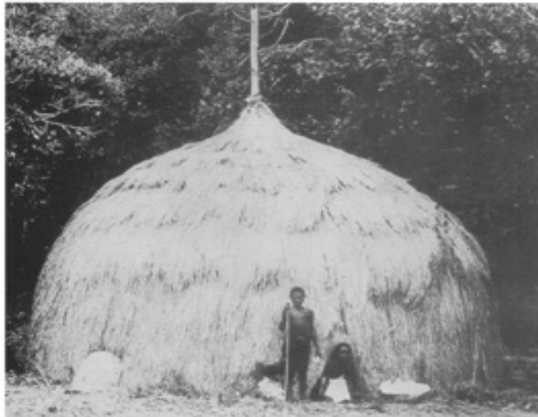
Figure 1.4 The Meriam people of the eastern Torres Strait Islands constructed pointed domes (skur mats) up until the turn of the 19th century, when their house styles underwent change under mission influences. A traditional medium-sized dome had an interior radius of about 2.85 metres and an interior height of 3.75 metres. Each dome accommodated a nuclear or an extended family. Construction was of (a) bamboo canes arranged in transverse arcs and tied together; (b) a clothing of leafy grass (impermeable) fastened with split bamboo lathen. (a) Photograph from the Australian Institute of Aboriginal and Torres Strait Islander Studies. (b) Photograph from Queensland Museum.
